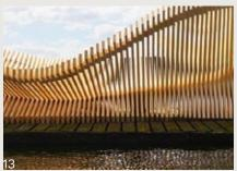
The upper and lower walkway railings can be united by creating a continuous ribbon railing that wraps across the bridge and is dramatically lit at night.
