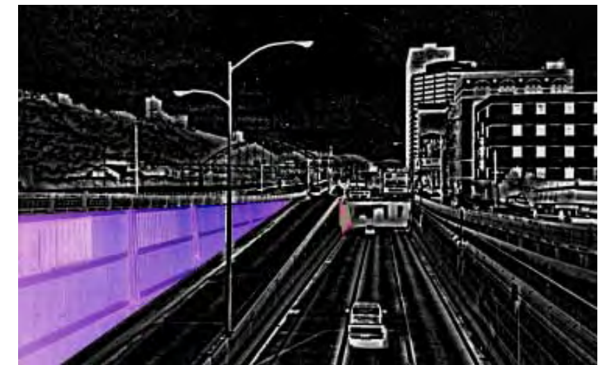
Acoustical panels help to mitigate traffic noise.
